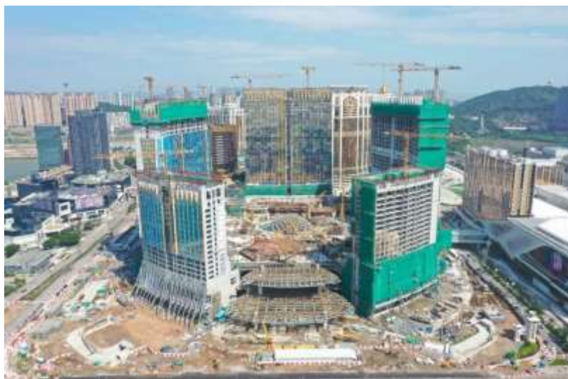
Latest photo of Cotai Phase 4 (November 2023)
